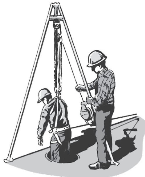
Illustration 3 | Retrieval Equipment in Use
